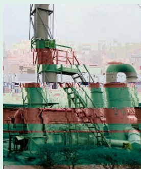
Waste Gas Treatment Equipment of the Sewage Tank—Dispose of Foul Smell of Sewage 污水池的廢氣處理設備 — 處理污水臭味
